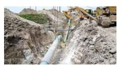
FIG 3. Laying Pipe for the Gulf Coast's new hydrogen pipeline. mercial and asset management to deliver value and continuous improvement to its Gulf Coast hydrogen customers. We anticipate an onstream date of early fall 2012. Here are the key milestones:
